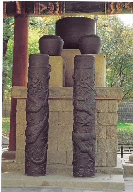
Automatically-striking clepsydra (自擊漏). Three reservoirs and two inflow vessels, now under preservation, 1536. Main reservoir (播水壺): outer diameter 93.5 cm × height 70 cm. Inflow vessels (受水筒): outer diameter 37 cm × height 199 cm. This characteristic Chosŏn period water clock with an automatic time signal apparatus was originally constructed by Chang Yŏng-sil (蔣英實) in 1434, then revised and reconstructed in 1536. Toksugung Palace.
