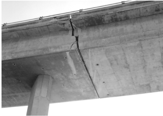
Pounding of Decks at Intermediate Hinge
