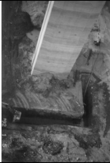
Pile Foundation Damaged by Fault Displacement
