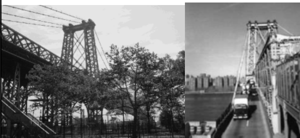
Williamsburg Bridge Open on December 19, 1903 (110 years)
