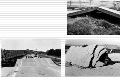
Failure of road pavement resulting from lateral spreading 1983 Nihon-kai-chubu, Japan, Earthquake
