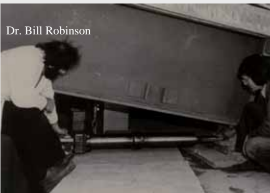
Lead Extrusion Damper
