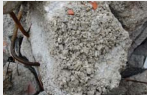
Failure of RC columns with poor concrete
