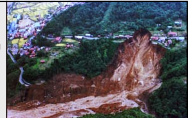
Failure Resulted from Slope Failure 1984 Nagano-ken-seibu Earthquake, Japan (M6.8)
