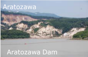
Damage Resulted from Failure of Mountains 2008 Iwate-Miyagi, Japan, Earthquake
