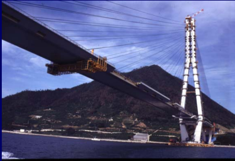
Tatara (1999) 270 + 890 + 320 (The Largest Cable Stayed Bridge)
